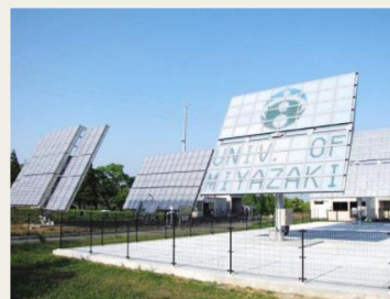
Sunlight tracking system
